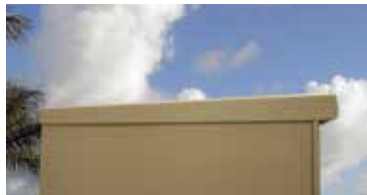
Sloped top for moisture runoff
